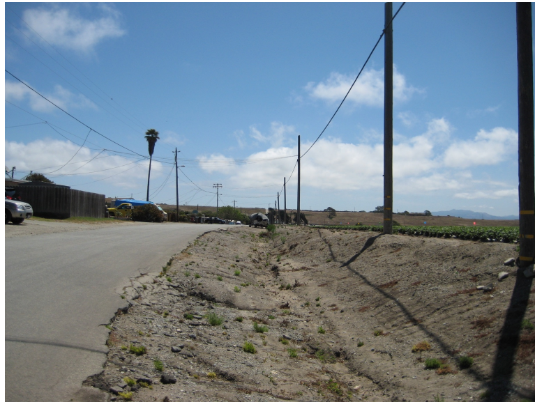
Struve Road. The community of Struve Road, located north of Moss Landing is currently receiving bottled water provided by the Pajaro Sunny Mesa Community Services District due to nitrate contamination of their drinking water well.
