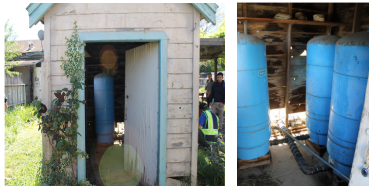
Figure 3 - Pump, Pumphouse, three storage tanks from the assessment trip. Located in the backyard of 742 Middlefield Rd.
