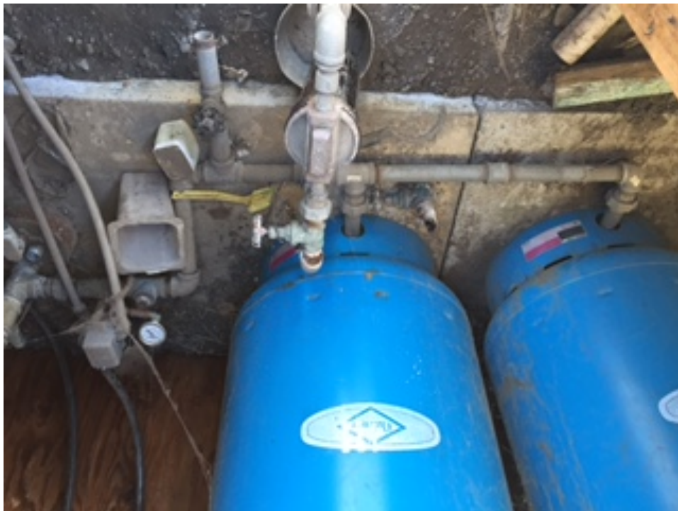
Photo 6 – Existing water system. Hudson Landing road
