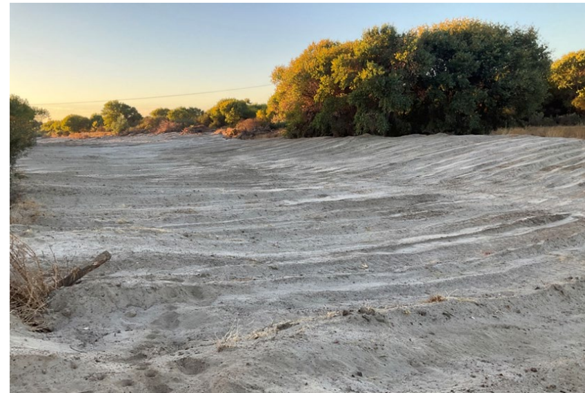
1.11b secondary channel (San Lucas) post-grading
