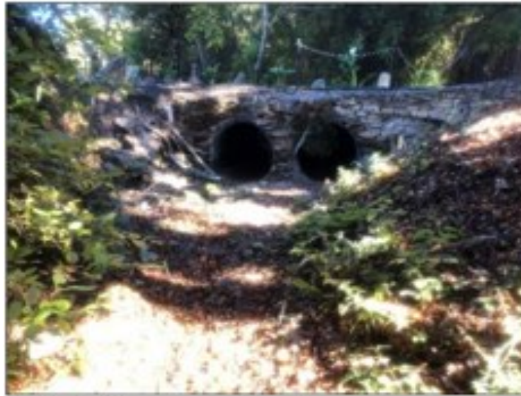
Before fish passage barrier removal
